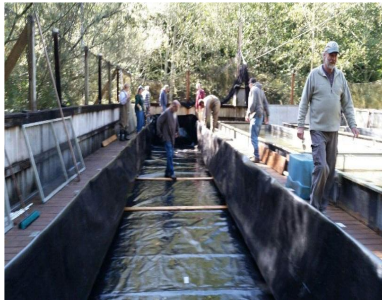
Raceway 3 New liner instillation Photo by Gary Underhill
